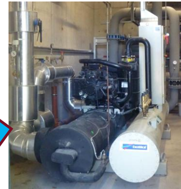
Cooling compressors
