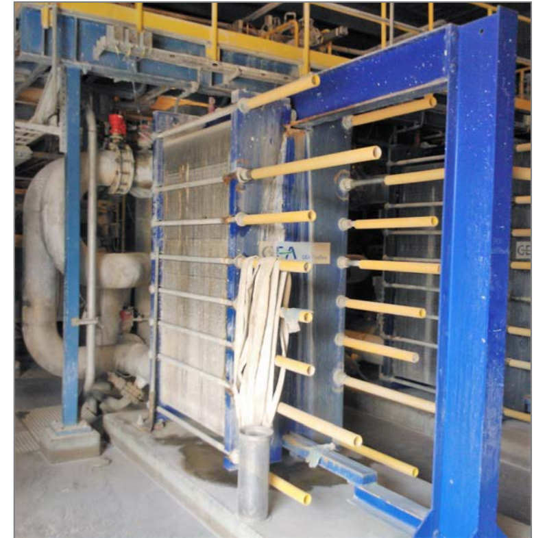
Rotary kiln (left) and plate heat exchanger (right) for recovery of flue gas excess heat to district heating at Portland Cement in Aalborg, Denmark. Photos: U. Persson.
